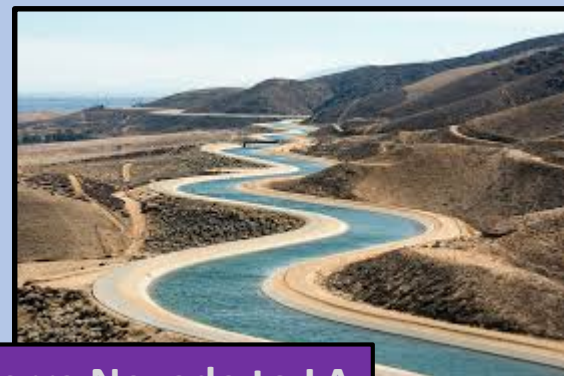
Sierra Nevada to LA Aqueduct
