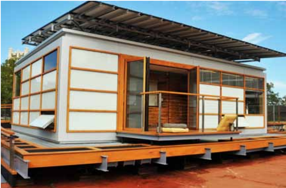
The Solar Roofpod on Marshak Terrace
