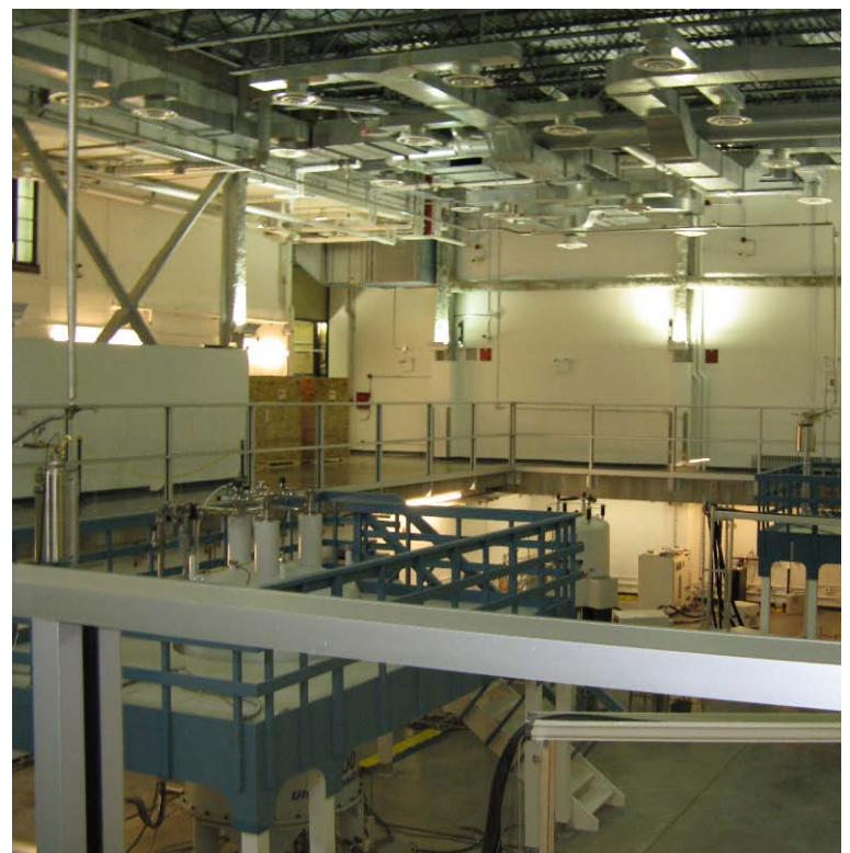
The catwalk overlooking the NMR's shows a very well maintained facility.
